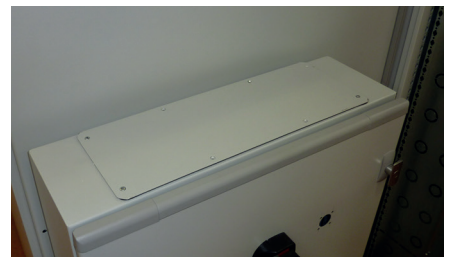
Standard IP 55 cable entry plate
