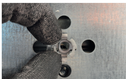
Remove the plastic cover at the rear of the enclosure and fit the clip-nut
