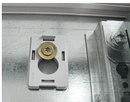
The keyhole shaped openings enable the cabinets to be attached and removed easily
