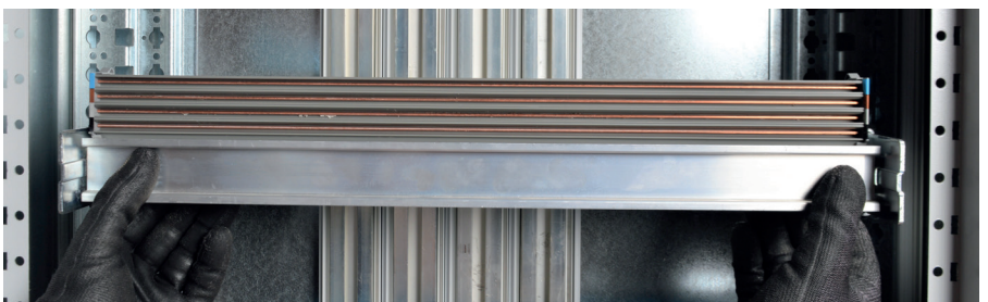
Position the rail in the enclosure in the up or down position.
