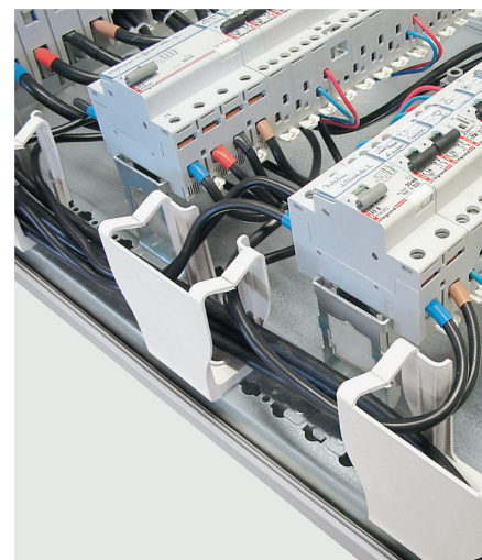
Example of wiring using guides
