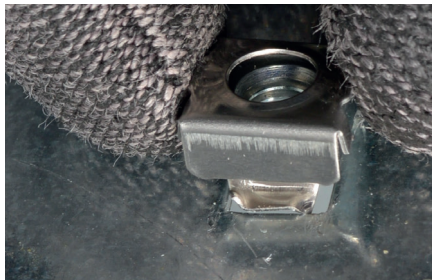
Fitting the cage nuts, via the rear of the metal plate.
